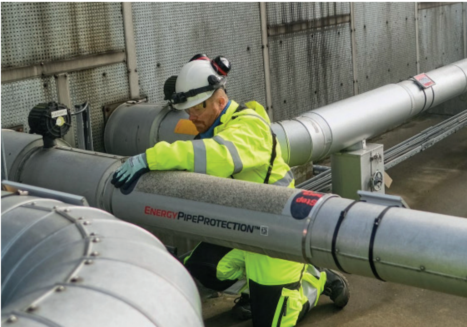
ENERGY PipeProtection™ protects cladding on insulated pipes
